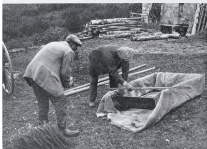
CONSTRUCTING A CORACLE from the body of an old dog-cart covered by a piece of tarred sacking. Bunches of broom bushes, seen in left-hand corner, are tied in the sacking to help keep the good ship afloat.
