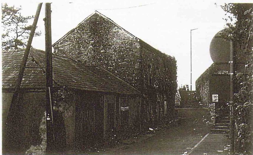
Dan-y-banc looking towards Castle Hill 2003 (Photo by Conwy Richards)
